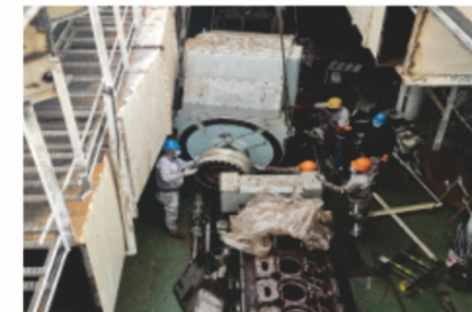
发动机拆解修复 Engine disassembly and repair
