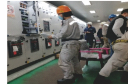
集控室修复 Repair of central control room
